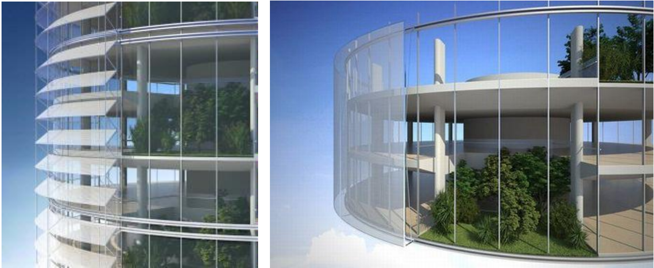
The external shading system sits like a skin on the outside of a building, moving around on tracks to shield the sun while still allowing daylight to penetrate. The sunshield is made from a lightweight frame incorporating photovoltaic cells.
